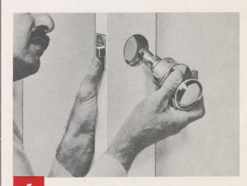
mounting strike, latch unit and lock in accordance with instructions packed with each lock. The result is a lock installation assuring years of trouble-free performance.
