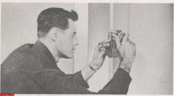
POSITION JIG ON DOOR—Insert backset guide into latch hole and press jig firmly against edge of door. Tighten adjustment knob on jig.
