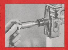
Insert the #932 hole saw into the pilot hole and into the backset guide. Cut halfway through door with hole saw, turn backset guide 180°. Finish boring from other side and door is now ready for installation of 5" backset lock.
