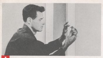
**REMOVE OLD LOCK** — Detach the old lock from the door, and remove the latch and strike plate.
