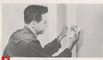
INSTALL NEW SCHLAGE LOCK—Slip the new Schlage lock in place. Connect lock mechanism to the latch mechanism and finish installation by installing inside rose, knob and new strike. The new lock fits like a glove.
